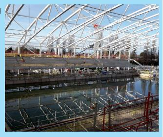
The 10m dive tower at the centre was completed earlier in the year and recent work has included the completion of the building facades. The roof is nearing completion and curtain walling and glazing is well advanced. Internally, high-level works within the pool hall have been ongoing, including pool hall lighting, fire alarm cabling and ventilation and heating duct work.
